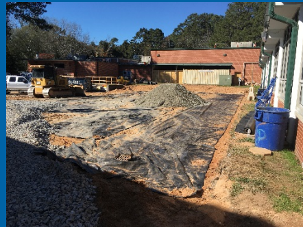
Installing GAB for Additional Parking and Laydown Areas
