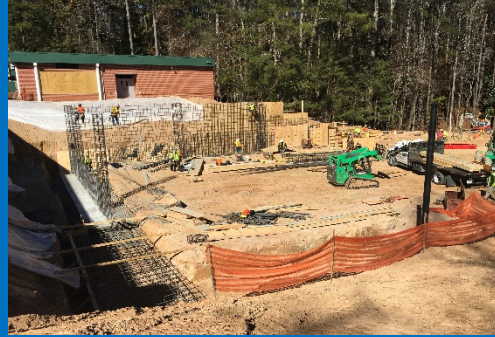
Reinforcing & Forming Walls at Gym Area
