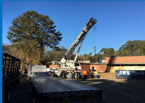
Crane Mobilized to Demo Existing HVAC Rooftop Equipment
