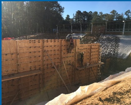
Rebar & Formwork at Gym Retaining Walls
