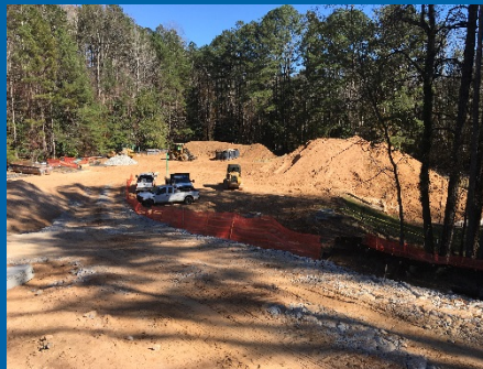
Stockpiling Soils from Excavation of Storm System
